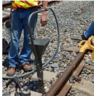
Injection Chute with Air Connection Mounted on Top of the Injector Tube
