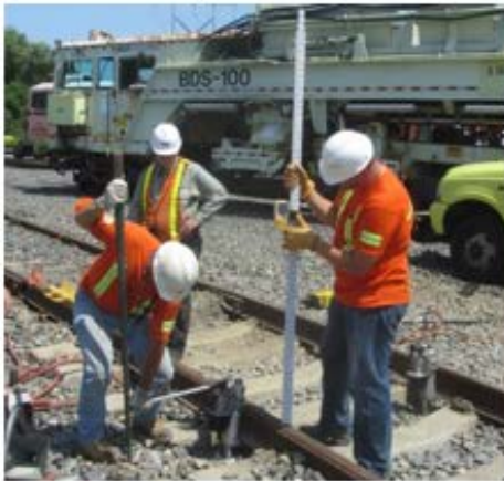
Surveying of Track to Establish Top-of-Rail Profile
