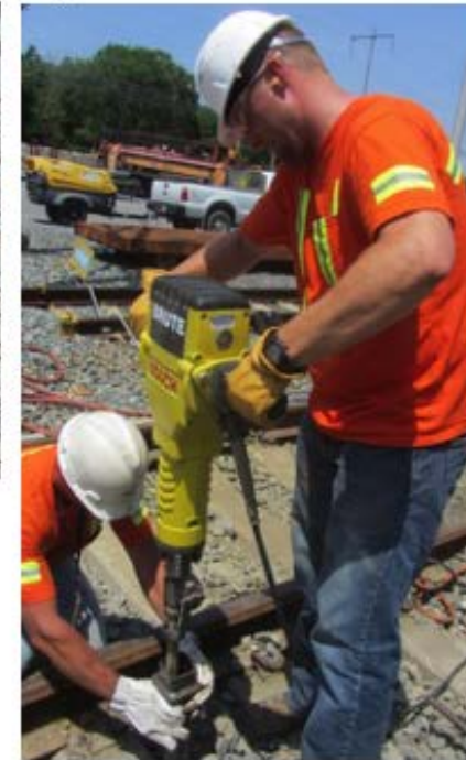
Driving Injector Tube Adjacent to Tie
