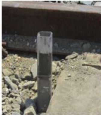
Injector Tube Driven Into Ballast Adjacent to Tie
