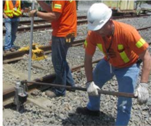
Jacking of Track to Pre-Determined Level
