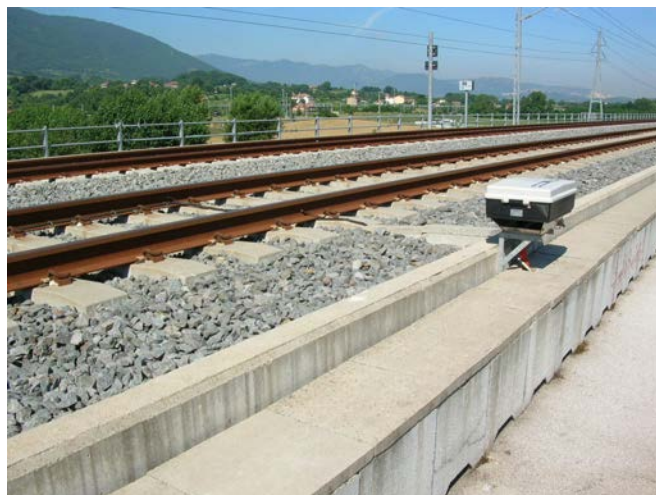
Figure 2 - Ballast profile lowered on the Rome-Naples HSL (Agretti, 2012)
