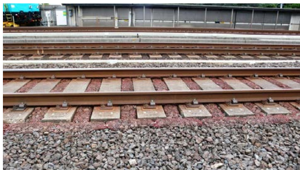
Figure 3 - Ballast Bag; the solution proposed in Japan (photo by T.C. Kao)
