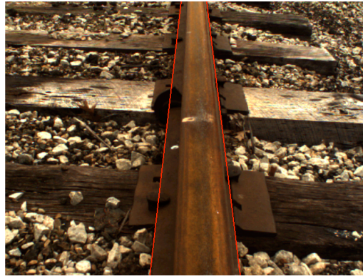
A: Delineation of the Base of the Rail from the Over-the-rail View Using the Strong Gradient Produced by the Edges of the Rail in the Foreground Against the Sections Containing Ballast and Ties in the Background
