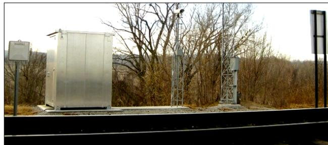
Figure 5: Southern view of the Sibley machine vision installation, showing from left to right, the AEI reader, equipment bungalow, camera, communication tower and exposure target
