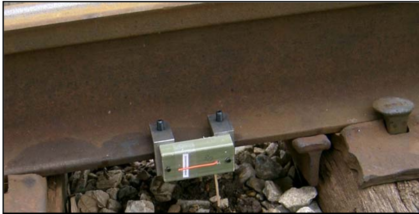
FIGURE 22 Sensor installed on a rail flange
