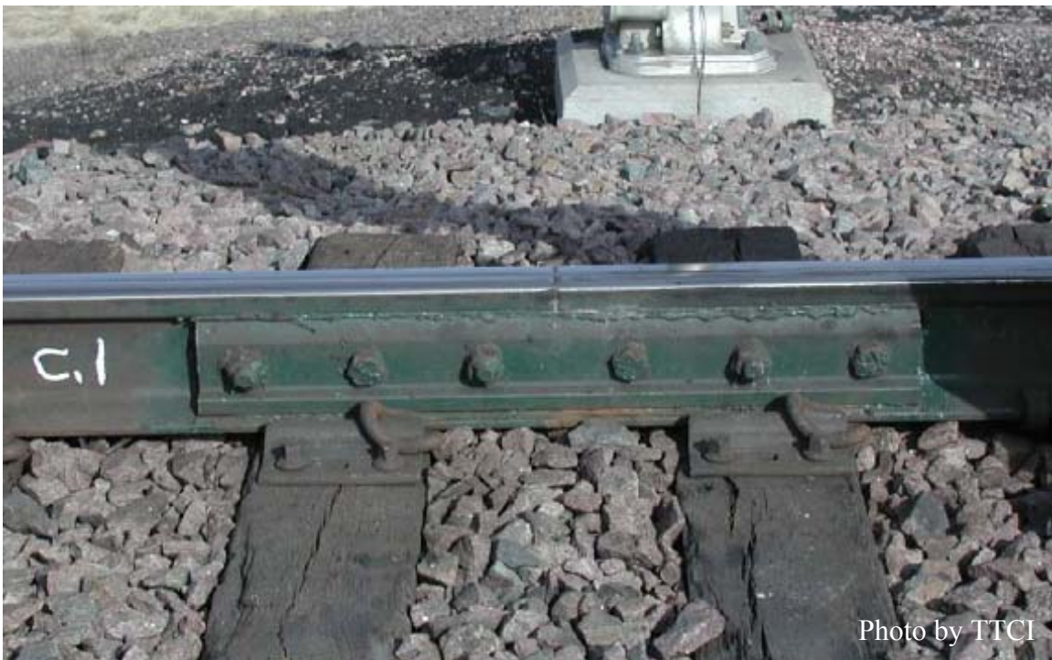
FIGURE 1: Typical Bonded Insulated Rail Joint
